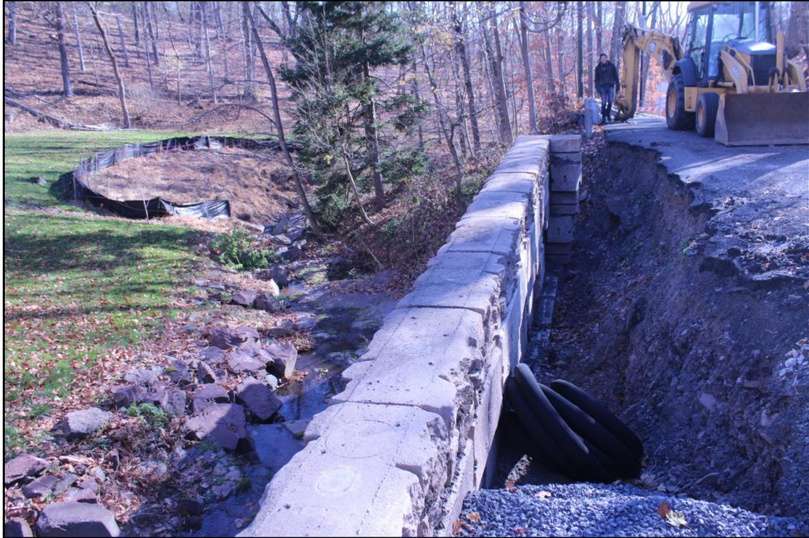
*Figure 7. Short Road under repair from scour damage at undersized culvert.*
