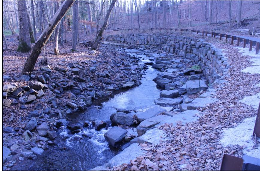
Figure 8. Fleecydale Road and its protection along the edge of Paunacussing Creek occupy a portion of the channel and may be the cause of erosion and subsequent armoring of the opposite bank.
