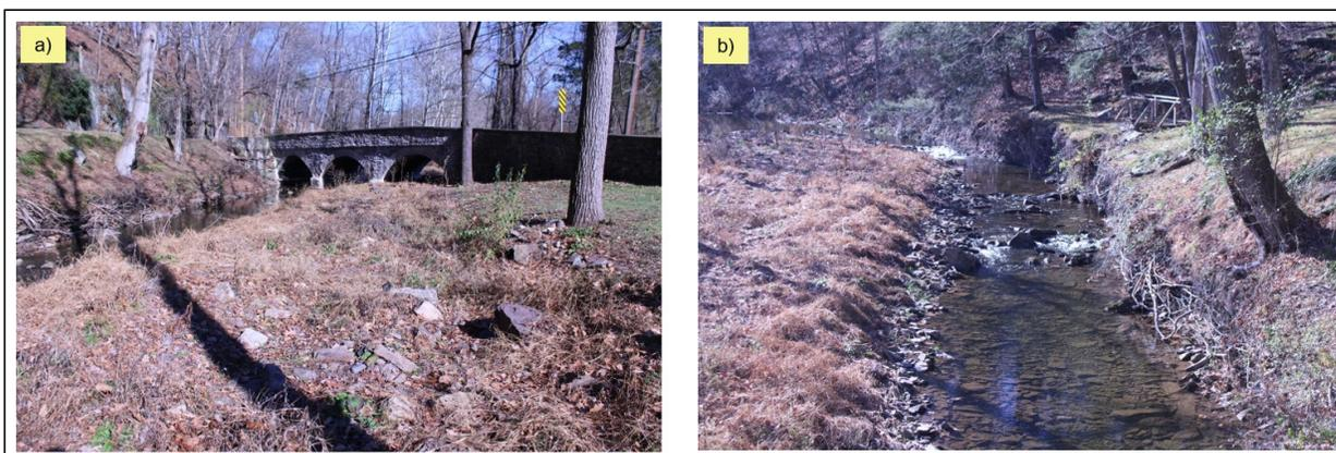
Figure 6. a) Triple-arch Fleecydale Road bridge with elevated road approaches blocking a portion of the floodplain may be responsible for b) deposition on the right bank (left side of photo) and erosion of the opposite bank.
