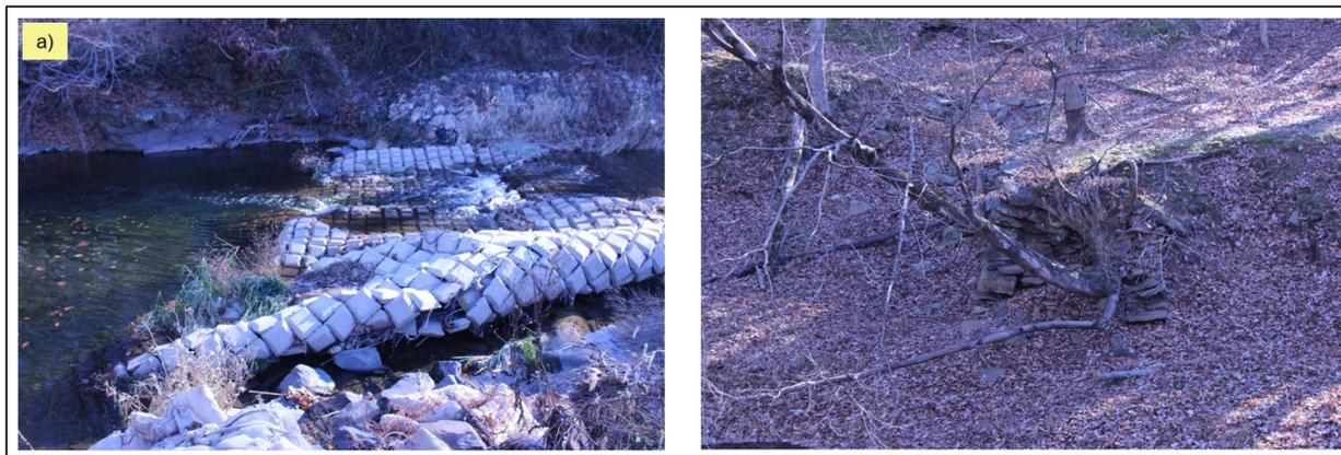
Figure 4. a) Erosion protection matting undermined at natural gas pipeline crossing immediately upstream of b) the remnants of a former mill dam.
