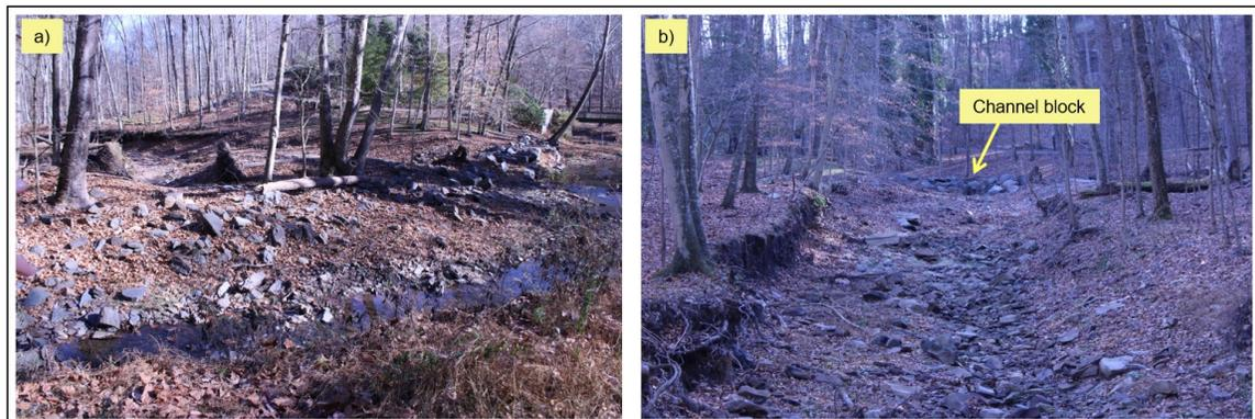
Figure 9. Constraints such as a) rock armor and b) channel blocks where no infrastructure is present divert erosive forces and may inadvertently add stress on infrastructure elsewhere.
